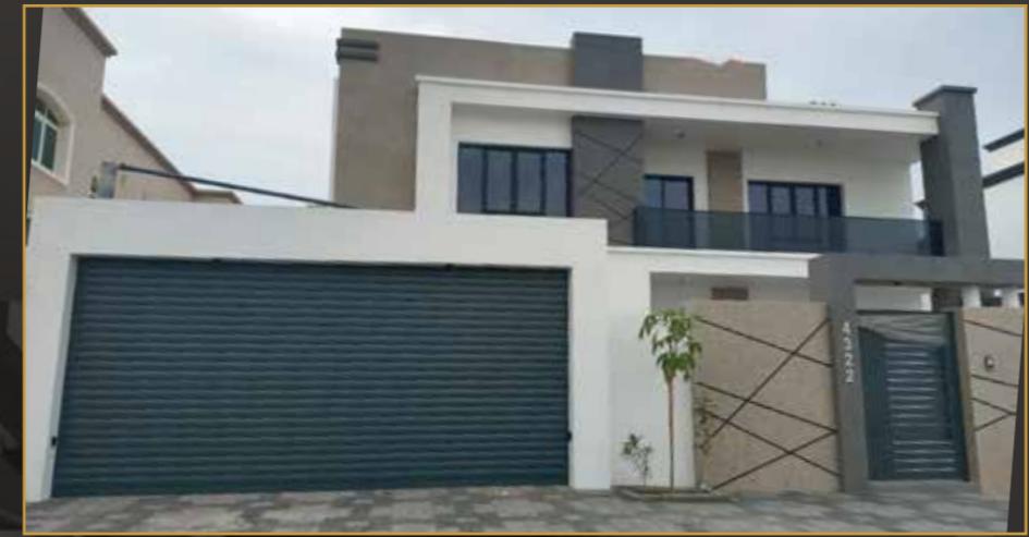
01 Private Villa Complex, Azaiba
