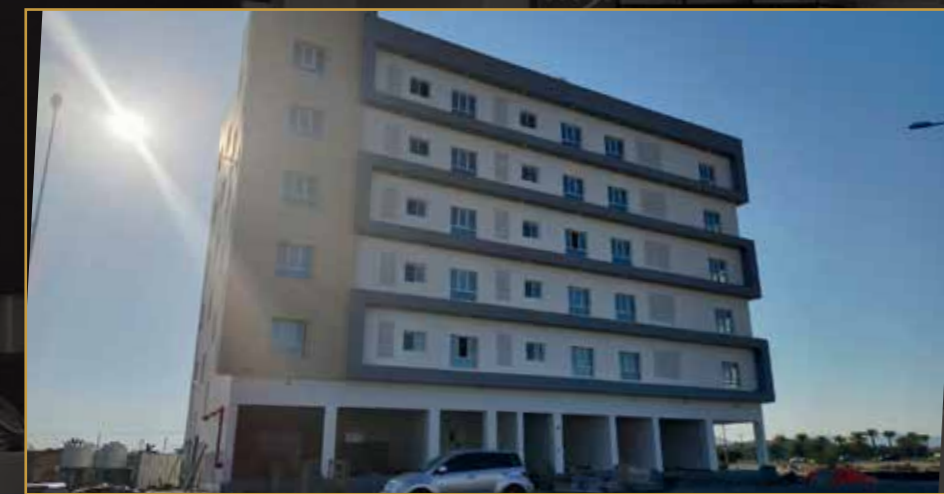
02 Residential Commercial Building, Mabela
